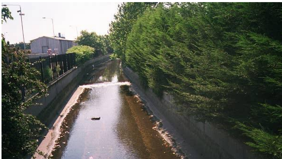
Plate C9: Enlarged (Overwidened) Cross Section
