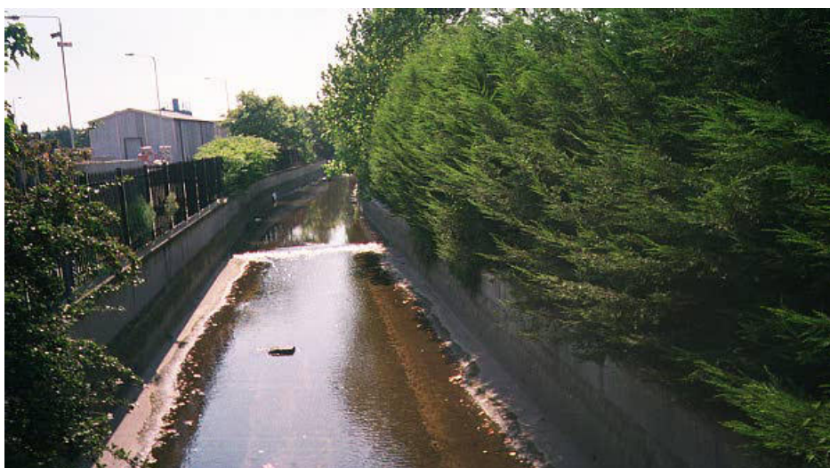
Plate C9: Enlarged (Overwidened) Cross Section
